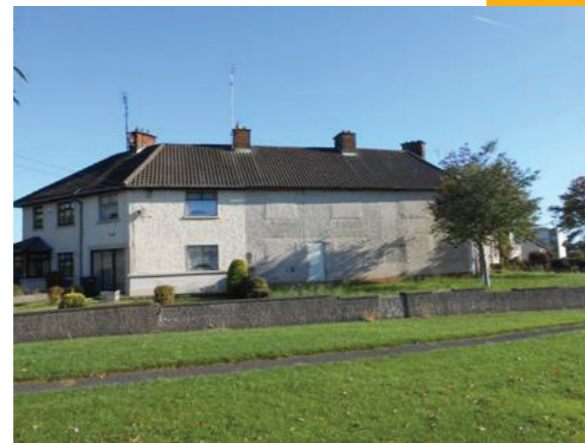
Bothar Brugha Before
